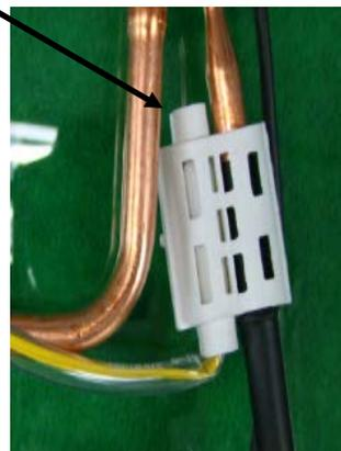
**The Sensor mounted correctly.**
